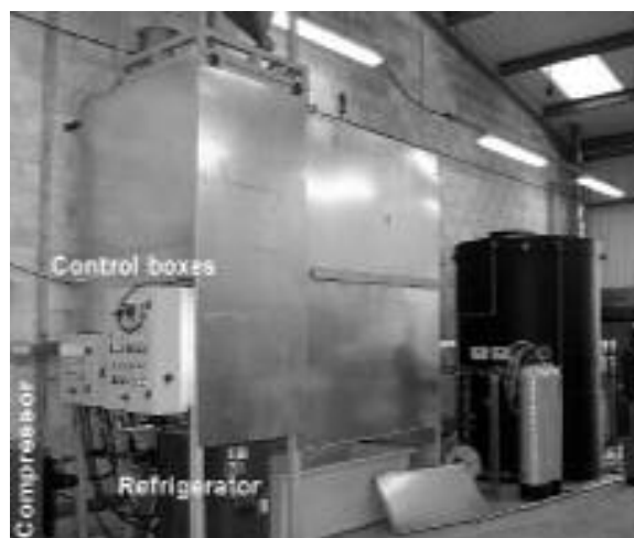
Figure 8: Process plant after cladding
