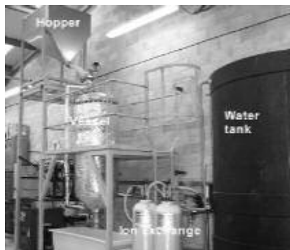
Figure 7: Process plant before cladding
